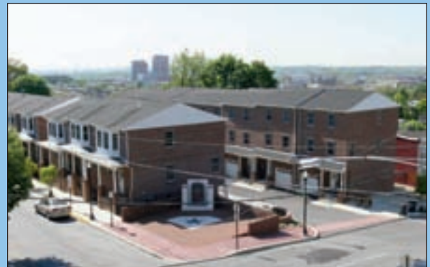
After meeting with the community, WHPartnership purchased a problematic market and additional homes on 6th and Franklin Streets in an effort to considerably transform this “at-risk” neighborhood. Franklin Chase is the first significant Hilltop homeownership development in decades – 19 new homes, all sold, emanating from the corner of 6th and Franklin Streets. WHPartnership is proud of the dynamic group of individuals that make up our Franklin Chase community.
